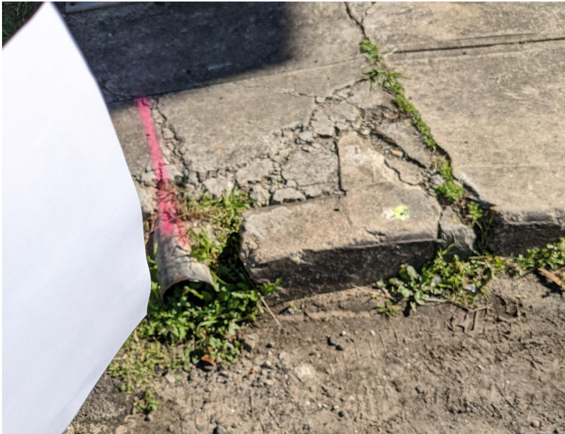
Photograph 2: 51 Drummond Street, Belmore NSW (26-08-2021) [Sealed surfaces around building exterior in moderate to poor condition]
